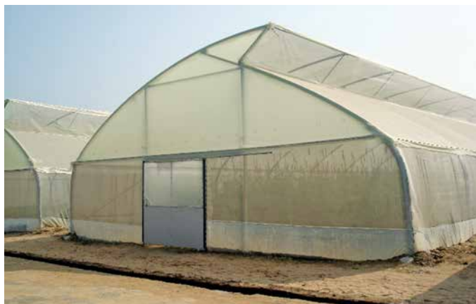
Open vent walk in tunnel
