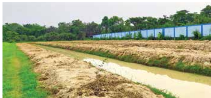
Dyke and canal preparation at low-land
