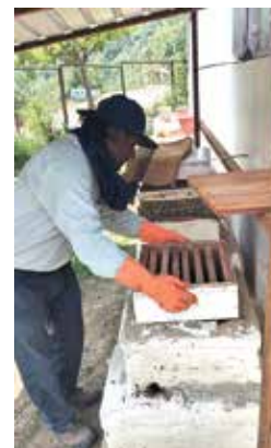
8. Installation of a super chamber over a mud hive
