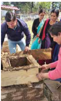
5. Removing the wooden frame the following day
