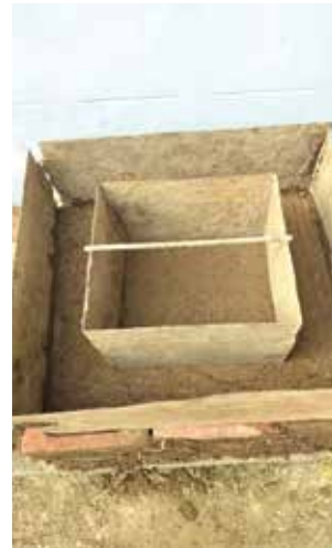
3. Positioning the iron frame onto the platform following the placement of a polythene sheet
