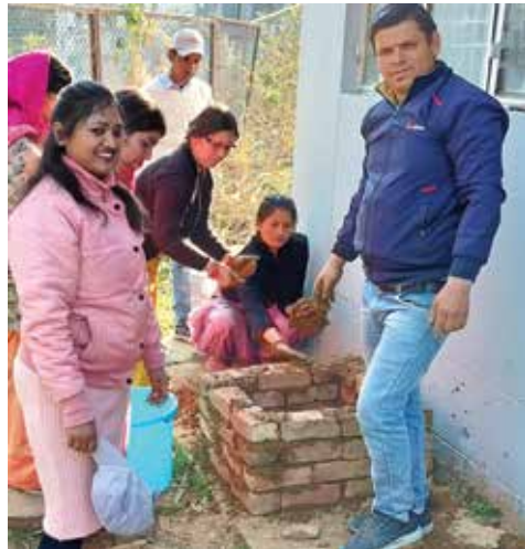
2. Construction of a platform using bricks
