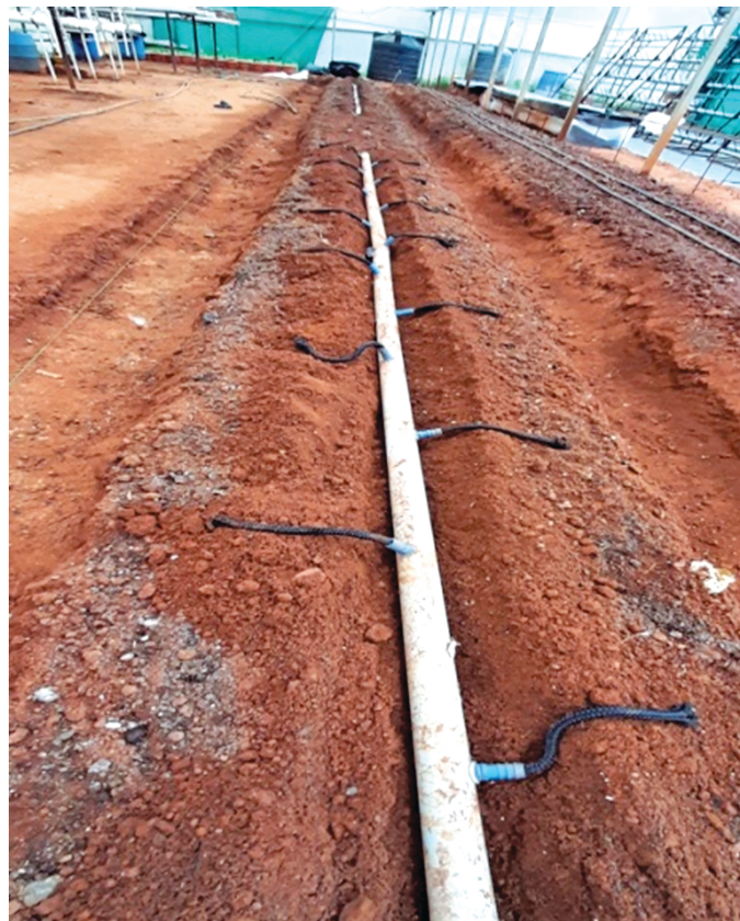
Wick system installation
