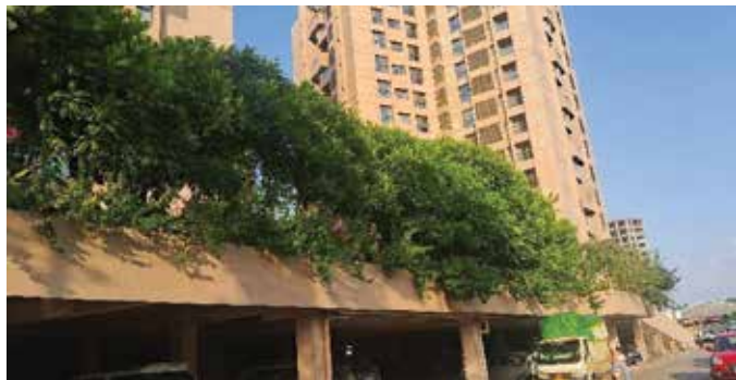
Intensive roof garden (Podium garden)
