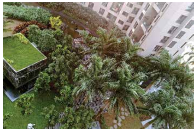
Intensive roof garden on a building
