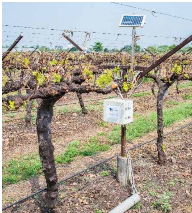
Sensors installed in a vineyard for monitoring vineyard micro-climate
