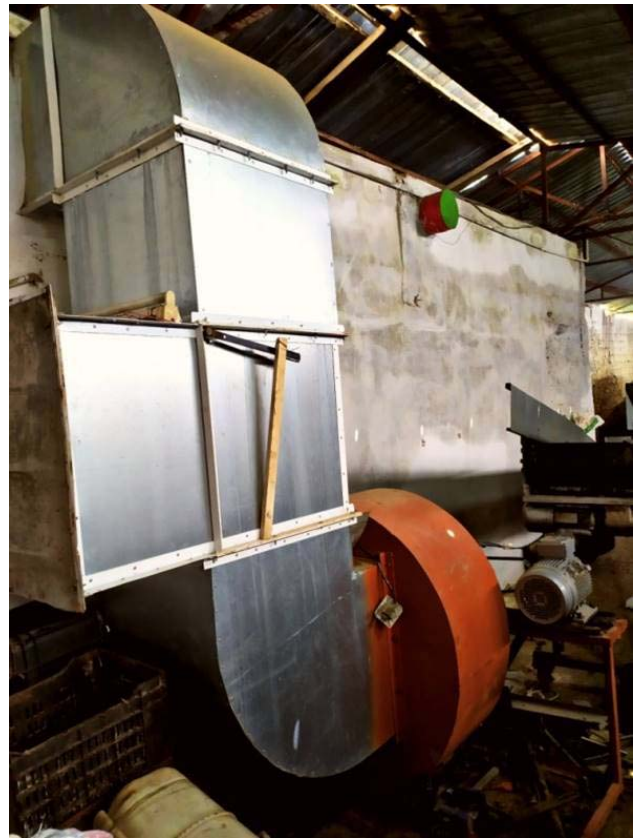
Fig. 3. Tool for processing compost into the pasteurization chamber
