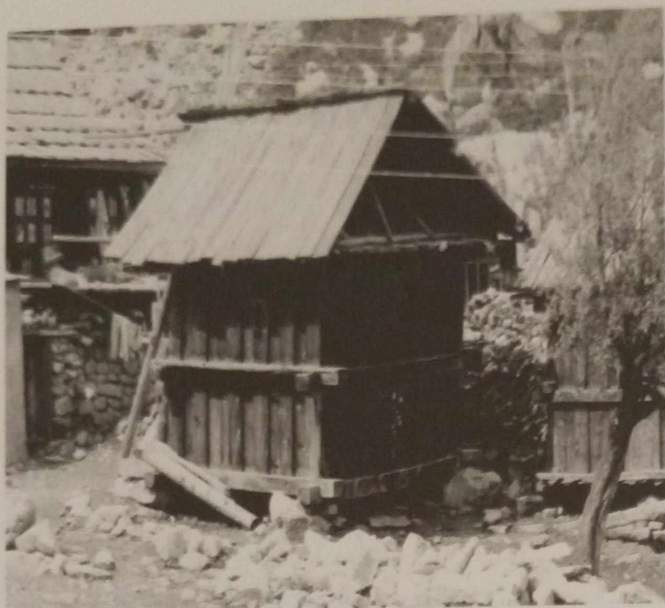
Fig. 1. Traditional seed storage structures ( kathars ) in tribal region of Kinnaur, Himachal Pradesh
